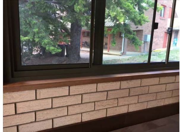
The new side windows from inside
