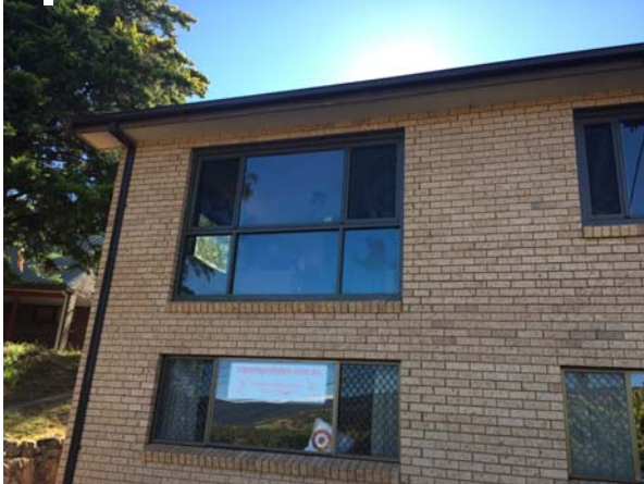
The new front windows from outside
