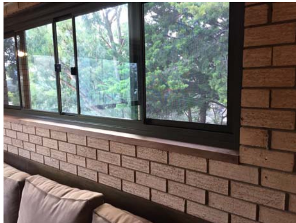
The new front windows from inside
